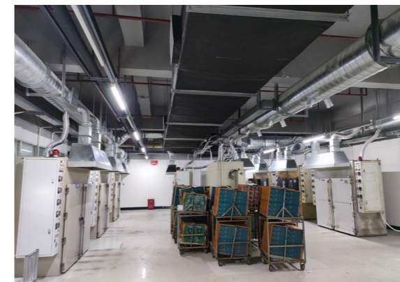
Waste gas absorption equipment inside the workshop and outside absorption tower of Multek China
