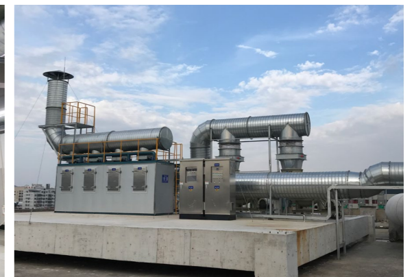
Waste gas absorption equipment inside the workshop and outside absorption tower of Multek China
