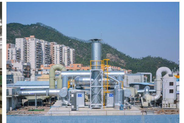
Waste gas absorption equipment inside the workshop and outside absorption tower of Multek Industries
