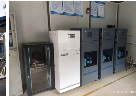
Industrial wastewater online monitoring device
