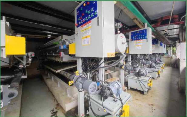
Upgrading of 8 high-efficiency filter presses to effectively reduce water content in sludge.
